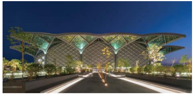
Haramain High Speed Railway Stations at Medina and Makkah
