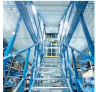
The movable high-bay storage unit stores a huge volume of goods in the smallest space possible
