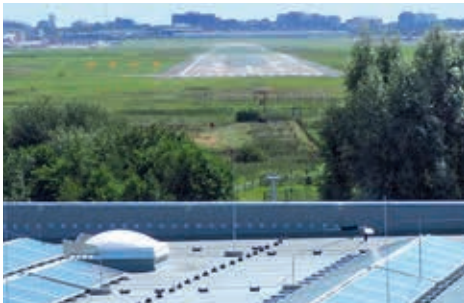
Photovoltaic system with a view of Hamburg Airport
